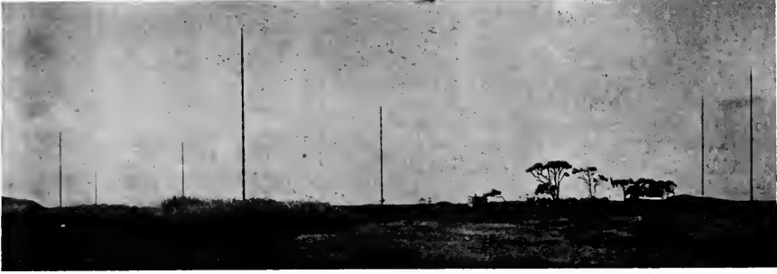
Marconi Duplex sending station, Kahuku, Hawaiian Islands. Messages are flashed to Japan (over 5000 miles) and to California (over 2000 miles) from this station simultaneously.
